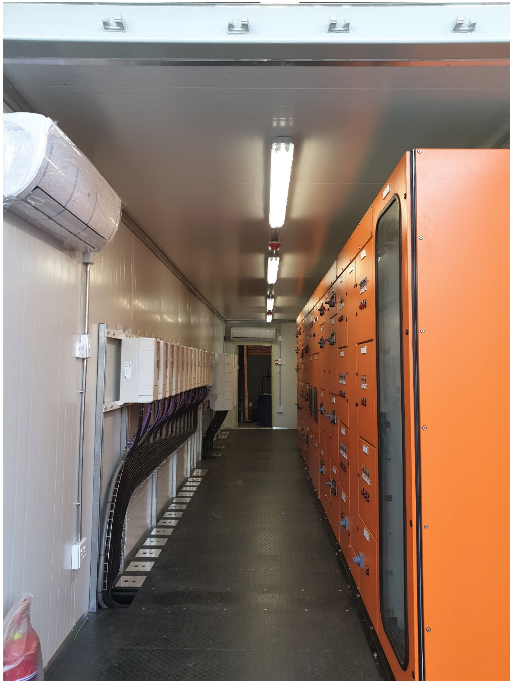
E,C&I DESIGN, INSTALLATION AND COMMISSIONING, NORTH MARA CONTAINERIZED MCC
