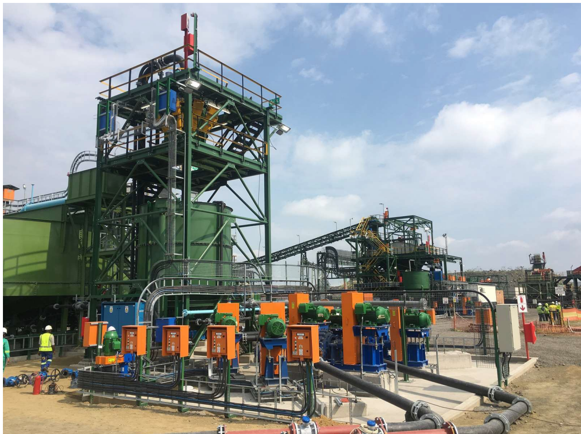
E&I INSTALLATION 4 TH STAGE CRUSHER PROJECT, THARISA MINERALS
