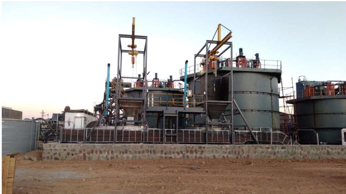
E,C&I INSTALLATION & COMMISSIONING, HASSAI GOLD PROJECT, SUDAN
