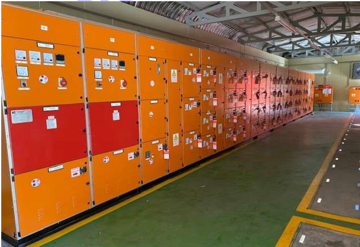
COMMISSIONING 351 MCC, ANGLO PLATINUM, RBMR, RUSTENBURG
