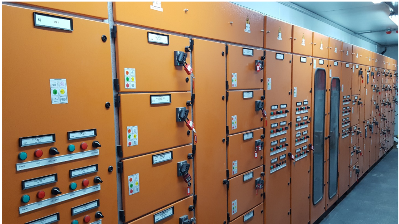
E,C&I DESIGN, INSTALLATION *& COMMISSIONING, CONTAINERISED MCC, SCOTGOLD, SCOTLAND
